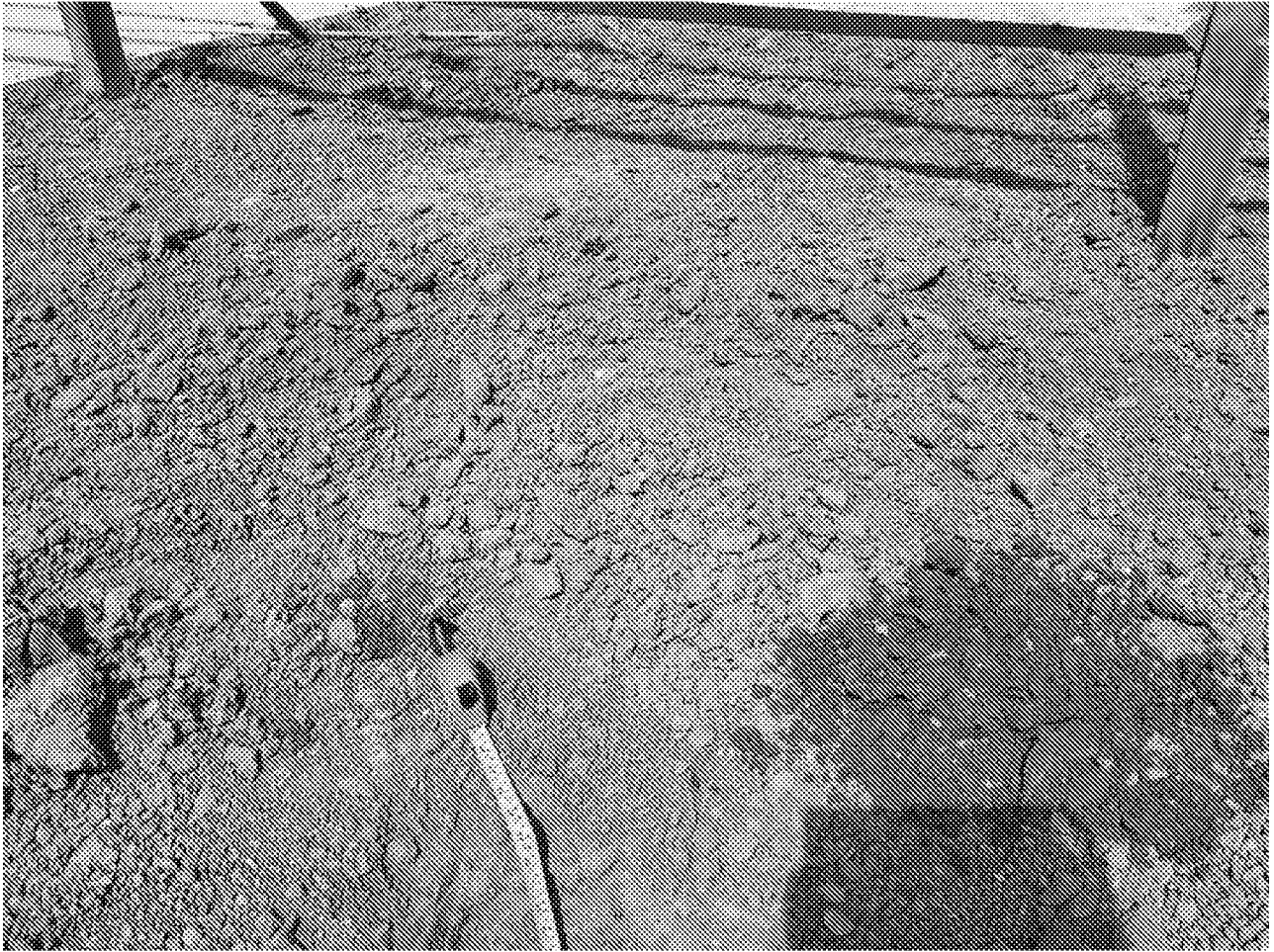
Photo of hole with tape in place
