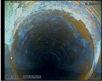
Observation [1]: Start Point: MH1
