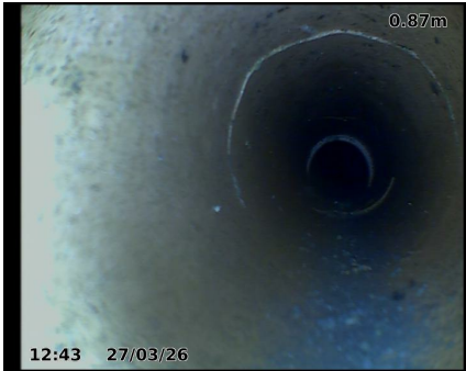
Observation [3]: CRACK
