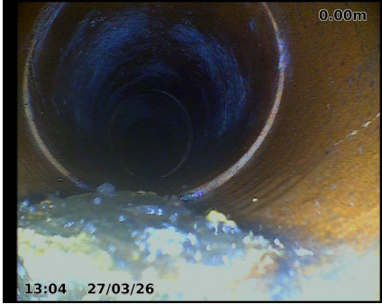
Observation [1]: Start Point: SWMH2
