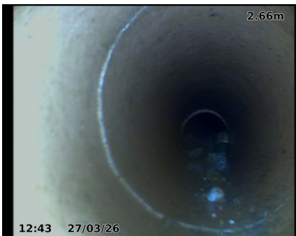
Observation [5]: CRACK
