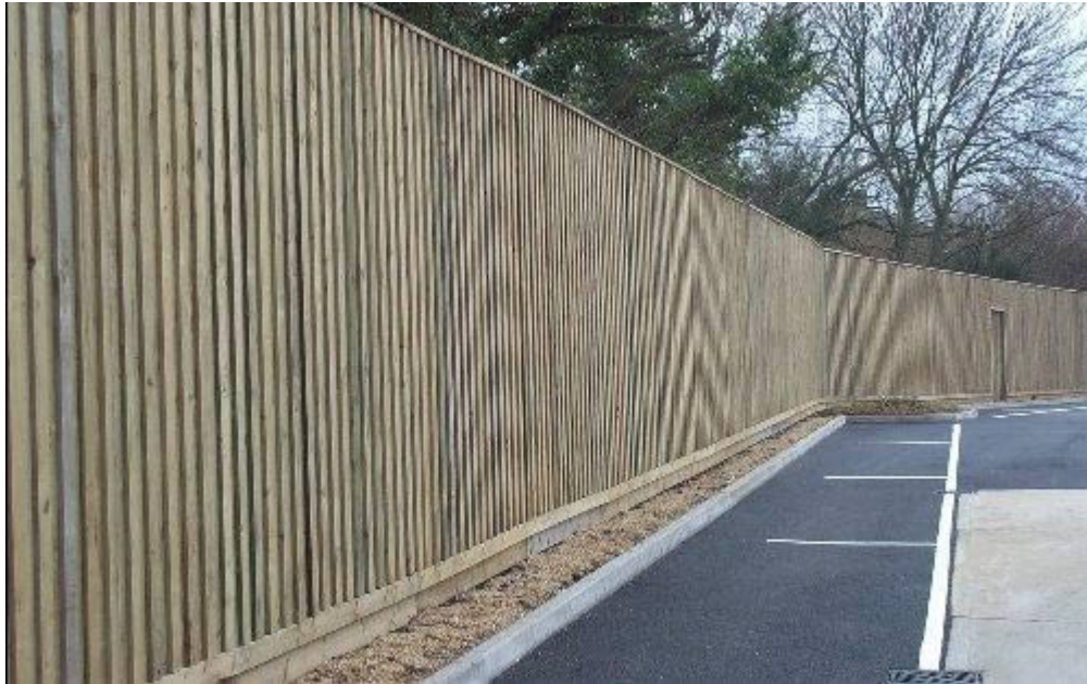
2000mm High Non- Climbable Vertical Boarded Acoustic Fence
