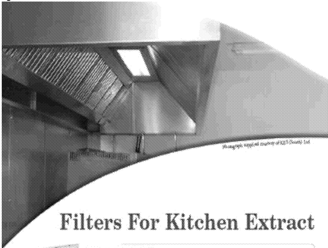
Figure 3: Hood Baffle Filters
