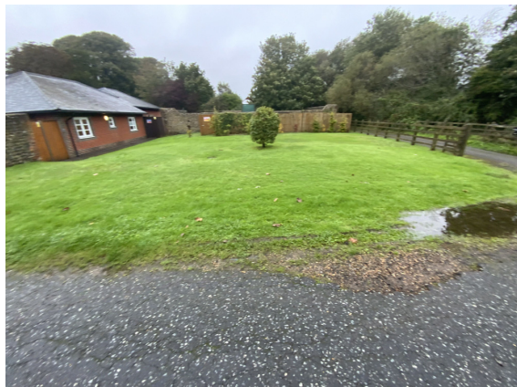
Estate style fencing
