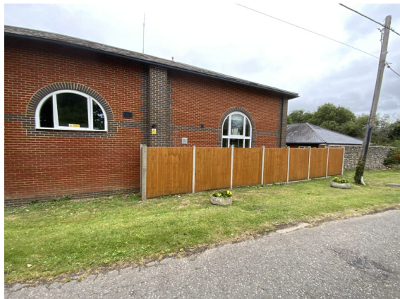
Existing close boarded fencing
