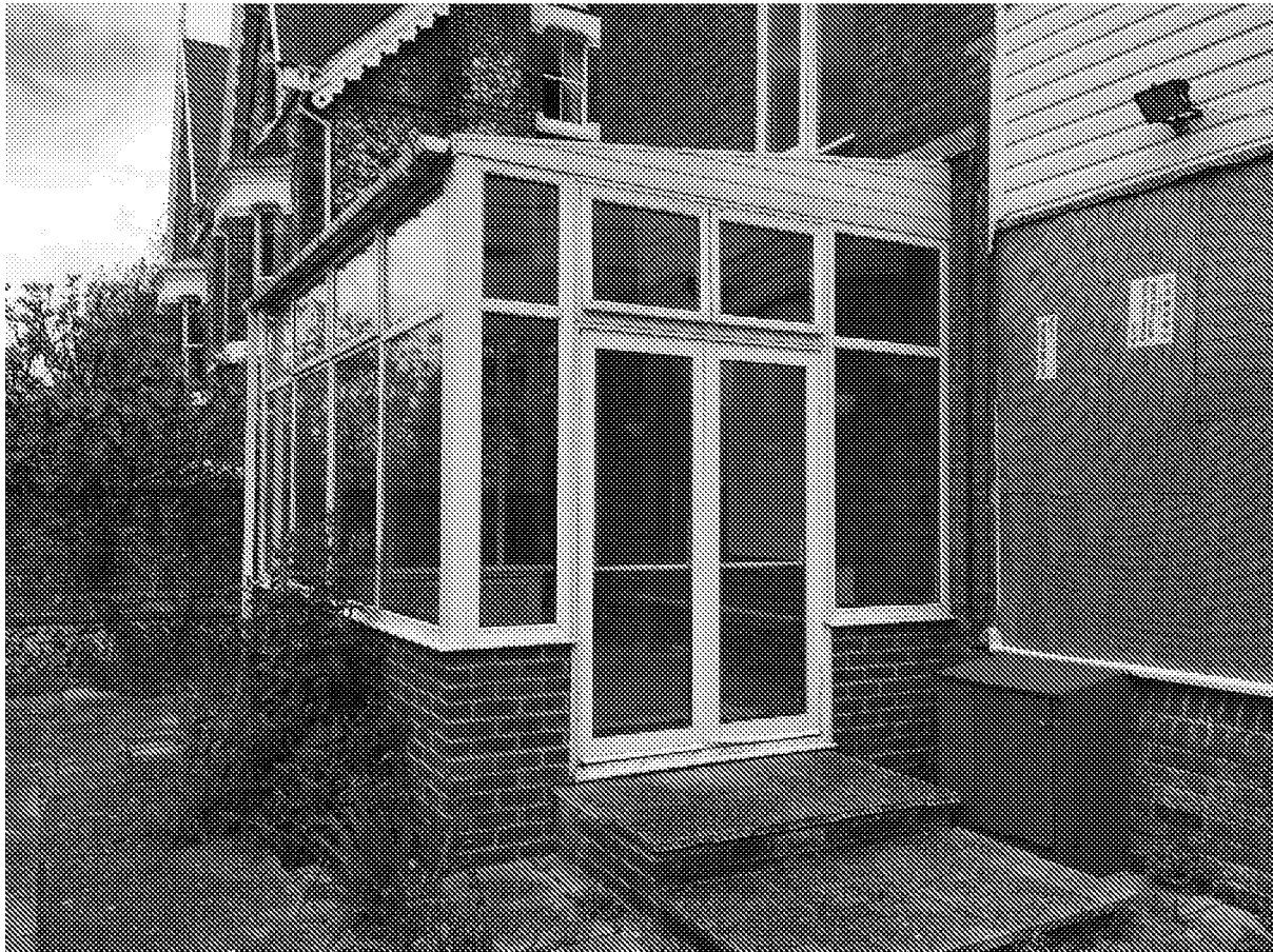
Existing non-original conservatory – proposed to be demolished.
