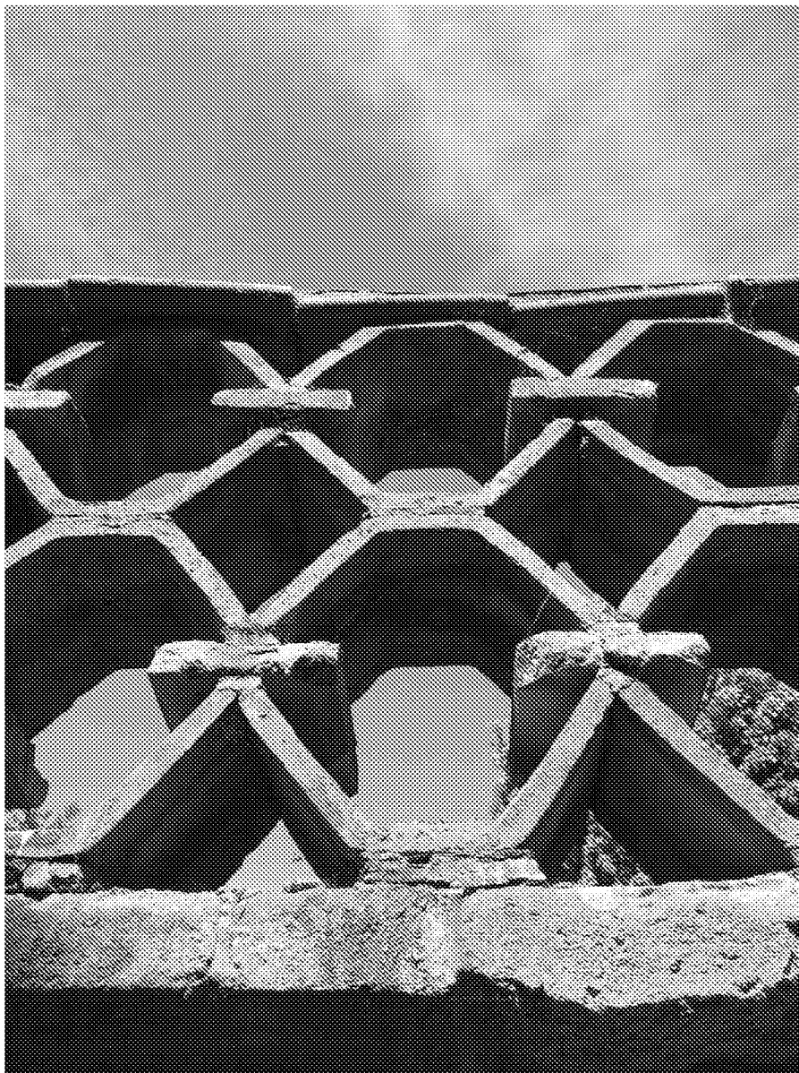
Original clay honeycomb walling
