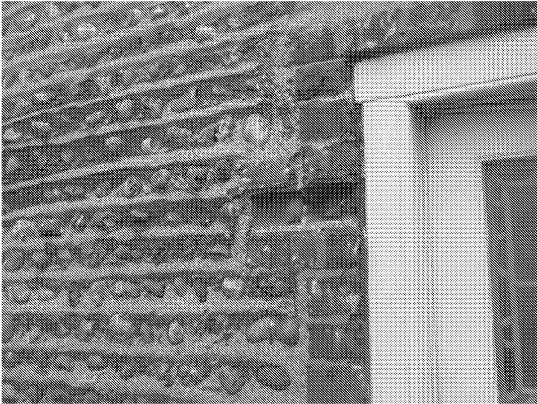
Damaged Brickwork
