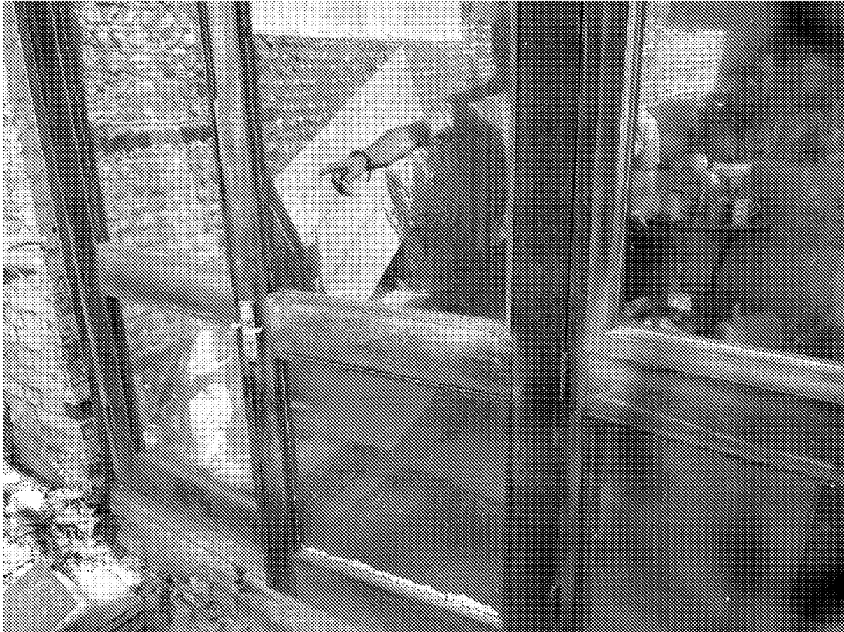
Timber rear doors.
