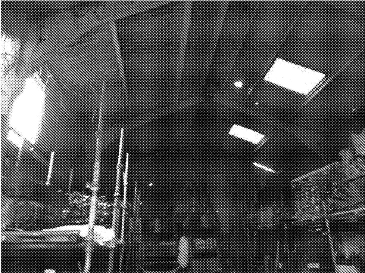
Figure 15. Internally the industrial shed is brightly lit by a window on the eastern face and plastic skylights.
