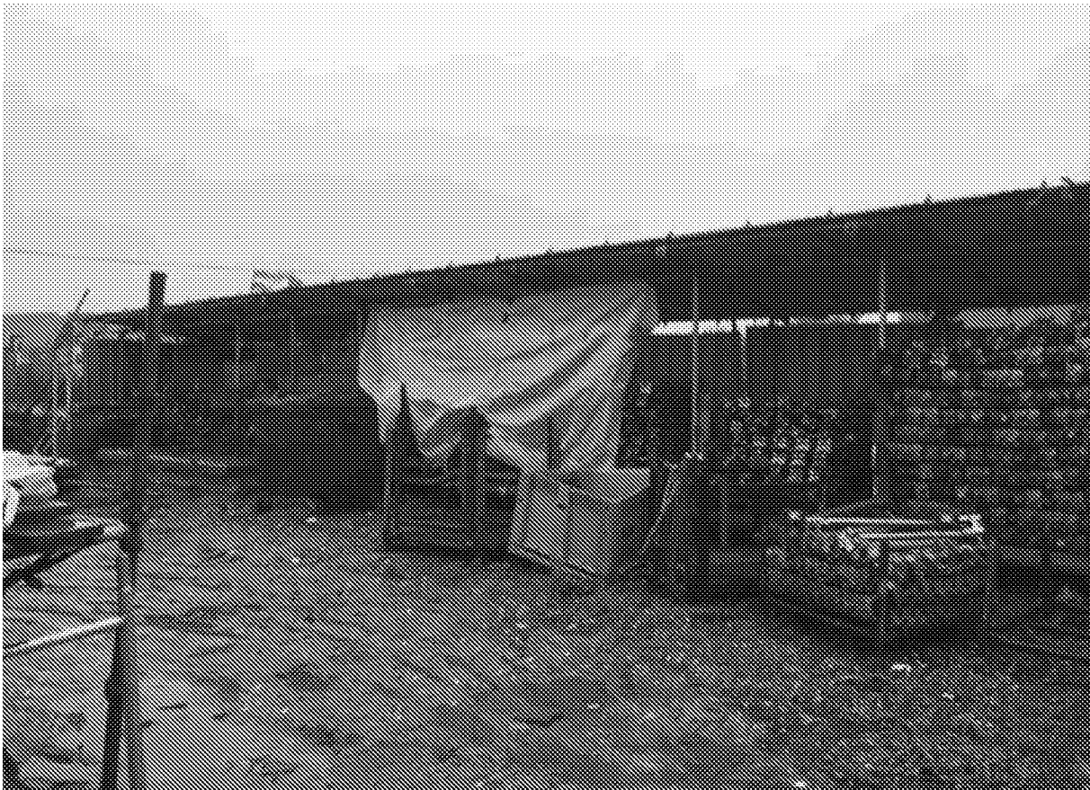
Figure 16. Open sided metal storage structures to the north of the industrial shed.
