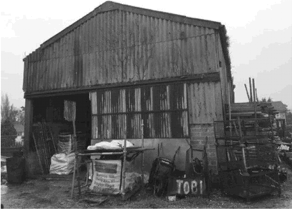
Figure 13. Northern face of the industrial shed used for storage with lower brick walls and an upper of single skinned corrugated chrysotile.
