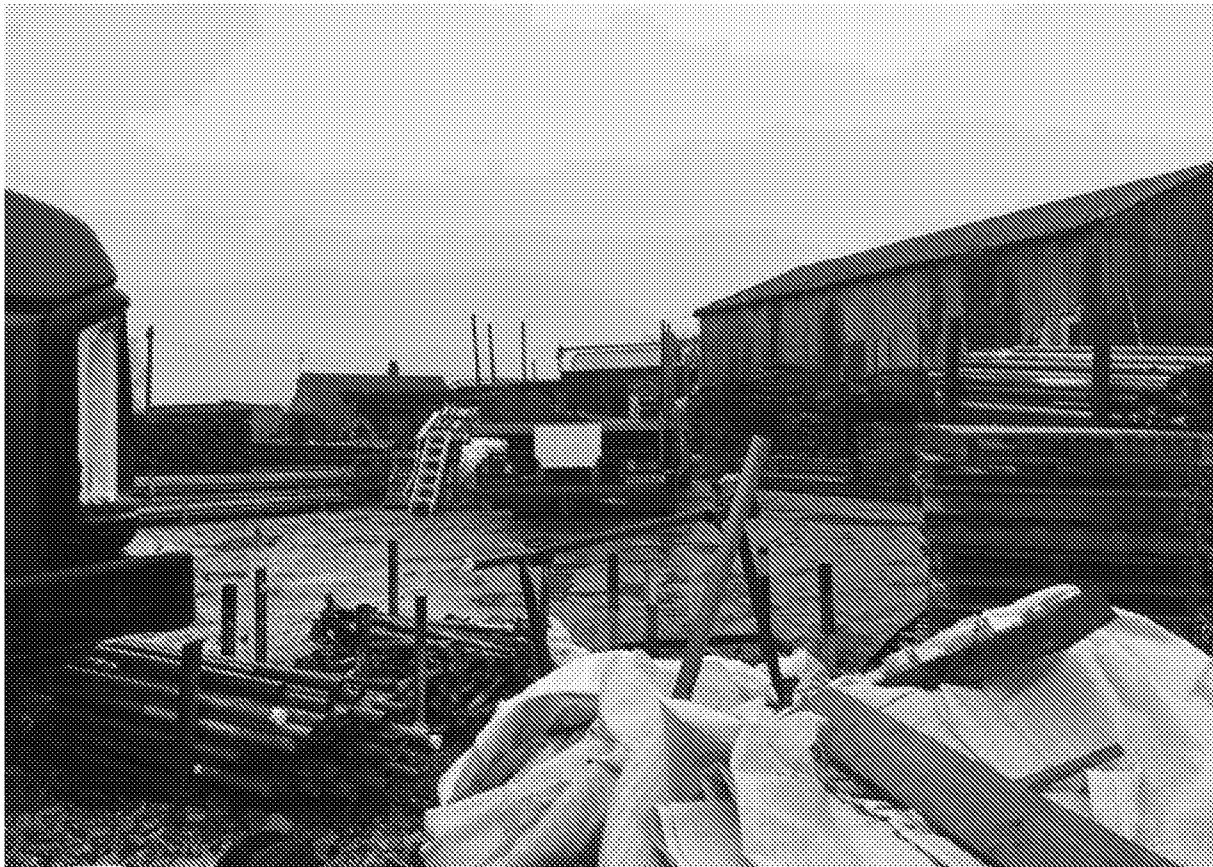
Figure 10. Bare ground area within the site's centre, where material and vehicles are stored.
