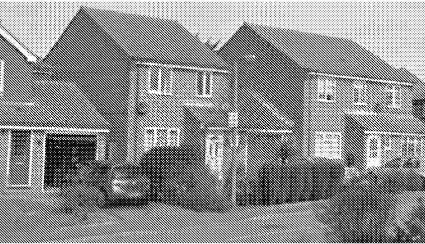
4. Housing development west of the application site
