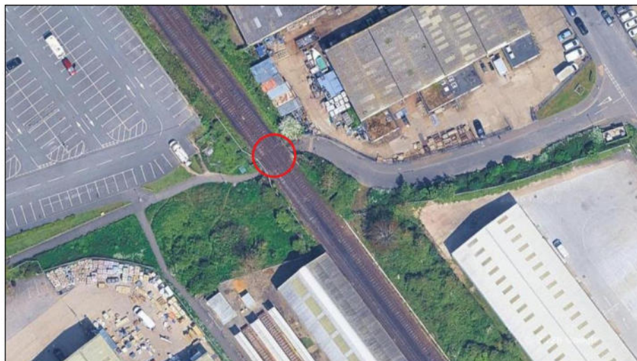
Figure 1. Aerial view of the Littlehampton Junction to Littlehampton Line with the location of the Cattle Creep Underbridge highlighted in red (Google Maps).
