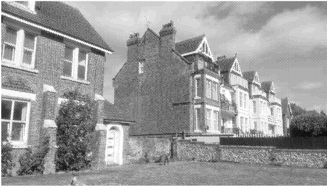
Figure 23: Side flank wall of 3, Irvine Road
