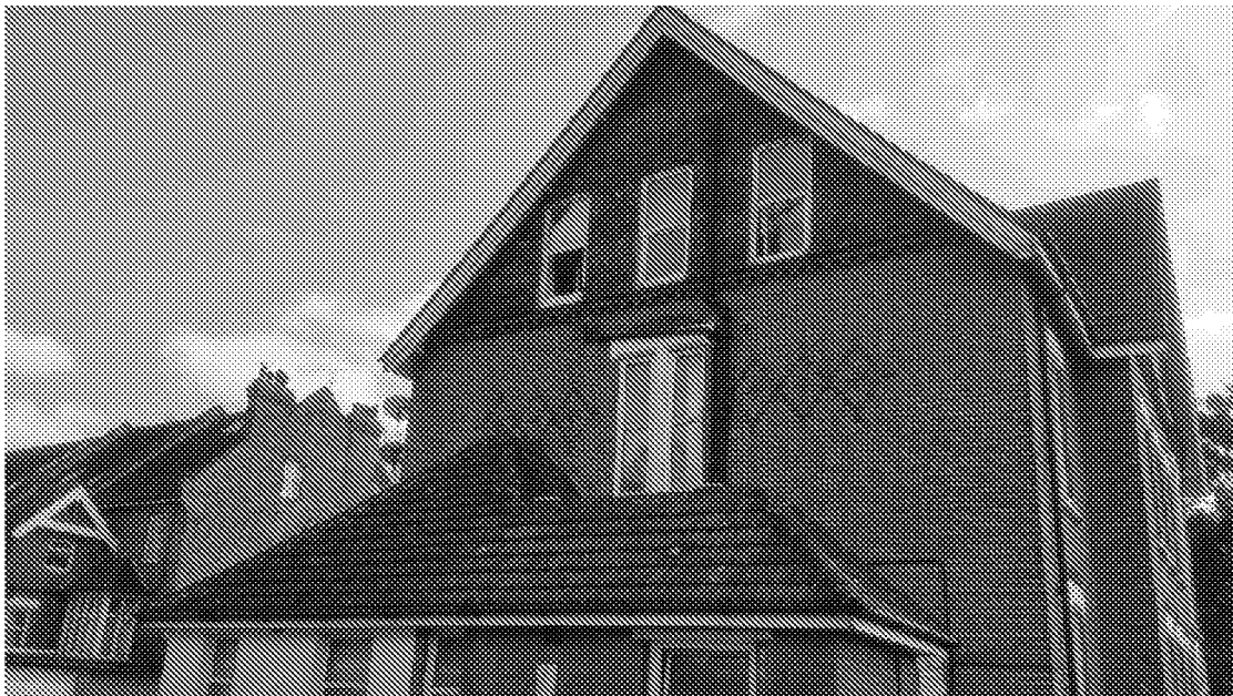
Figure 17: End elevation of Wellesley Court. The proposed new block picks up on the various elements on the building.
