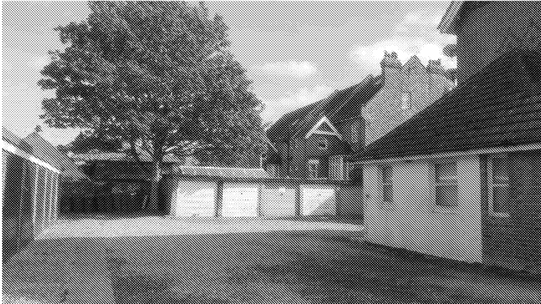
Figure 16: Five lock up garages on eastern boundary, to be demolished. The tree would be retained.
