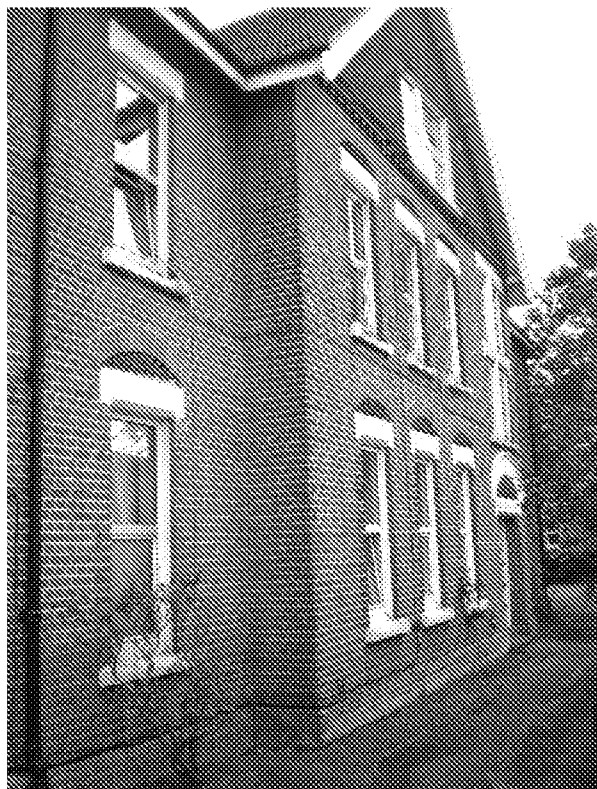
Front (West) Elevation of Wellesley Court with a central gabled projecting bay. The entrance door and main staircase compartment are offset. This is the principal elevation. Low Heritage Significance but important in the local context.
