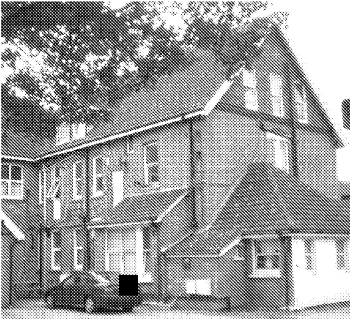
The rear (east) elevation of the west wing, showing the circa 1912 - 1938 lean-to extension with a wide window and a smaller, later lean-to extension to its north (right).
