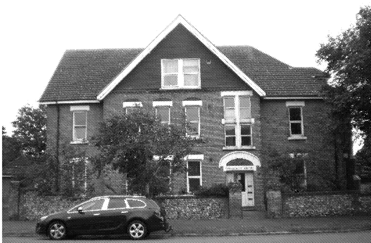
Front (West) Elevation of Wellesley Court with a central gabled projecting bay. The entrance door and main staircase compartment are offset. This is the principal elevation. Low Heritage Significance but important in the local context.
