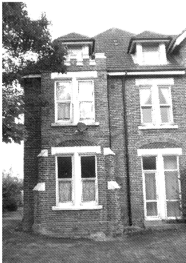
Projecting window bay with crenalated parapet. Satellite dish – harmful modern alteration.
