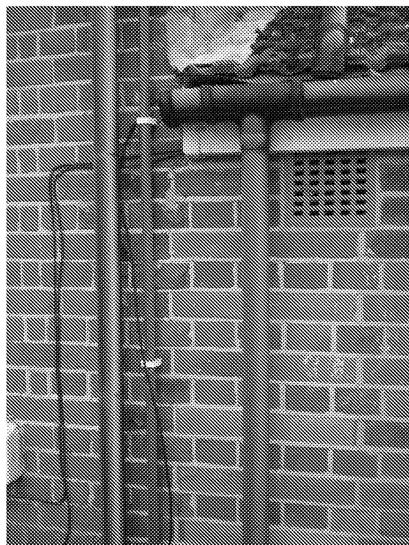
Join in brickwork between the 1912 – 1938 leanto extension and the later smaller lean-to extension.
