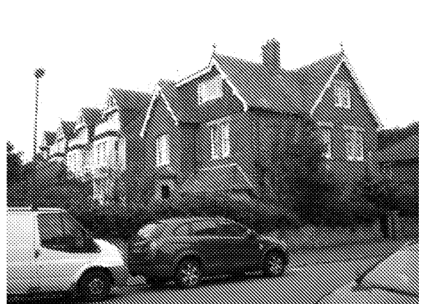
3-5 Irvine Road. Three-storey late Victorian townhouses, converted to flats - Low Heritage Significance. Brickwork painted and balustrading - unsympathetic modern alterations.
