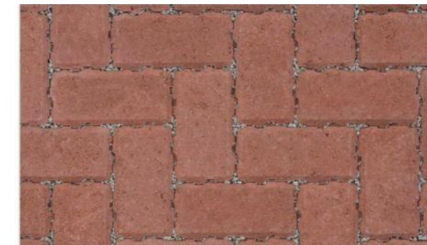
4. NEW PERMEABLE RED PAVING
