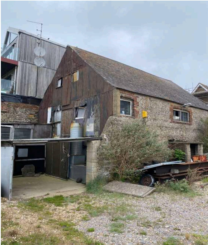
Photograph 7: The existing garage on Site, facing northeast. Neighbouring residential land can be seen adjacent to the garage.
