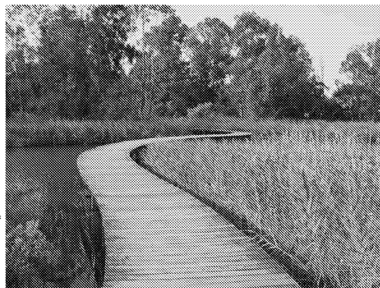
Walkway within wetland
