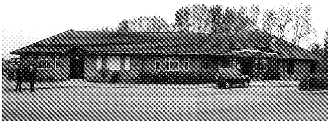
Existing school building
