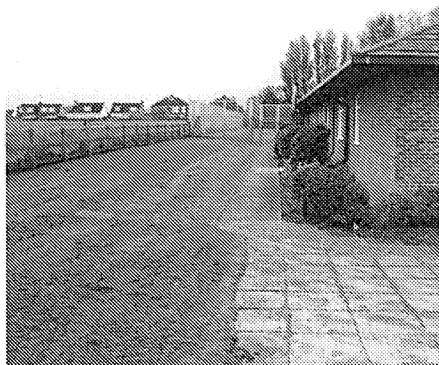
Site of extension looking west
