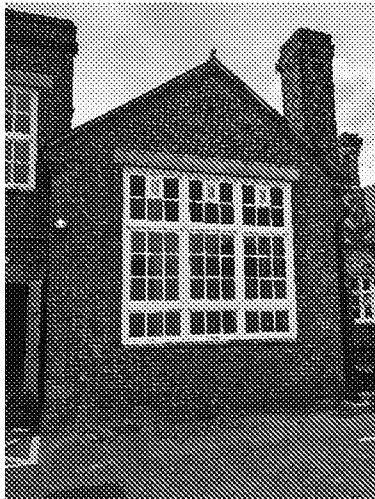
Figure 4 -- Toilet block Externally
