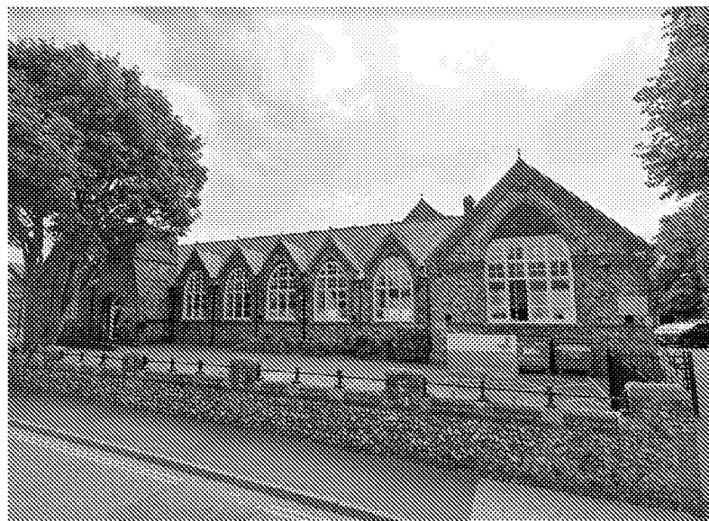
(Figure 1 – WSCC APC/ East Street School as seen from East Street)
