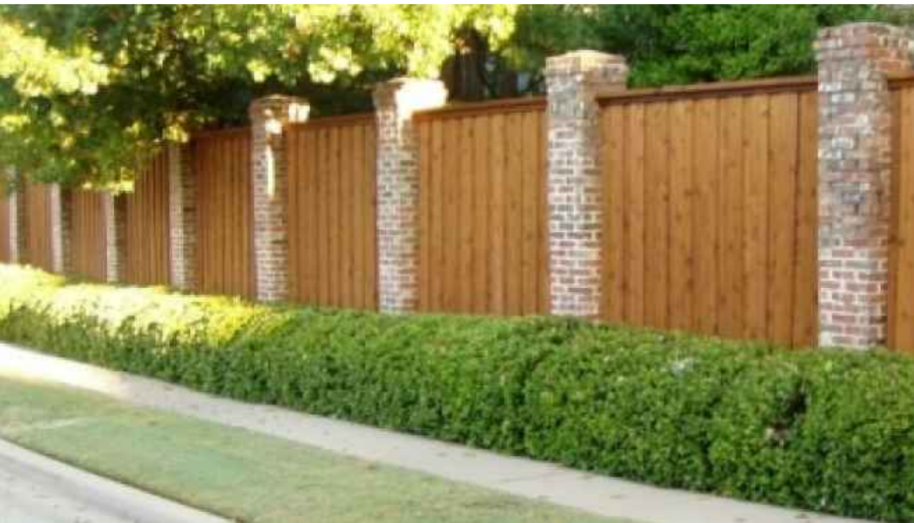
Brick piers and timber infill fencing
