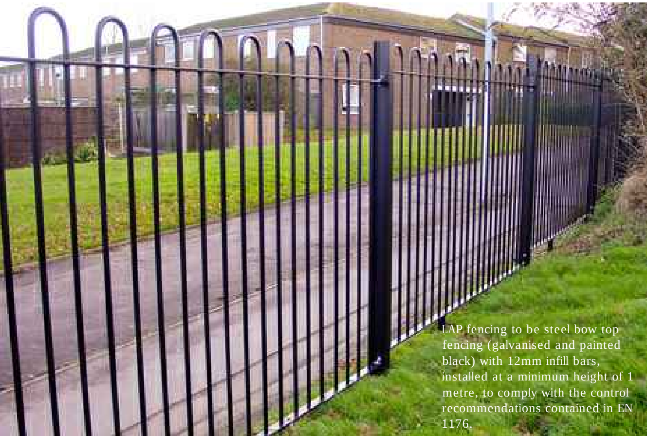
Steel bow top railings
