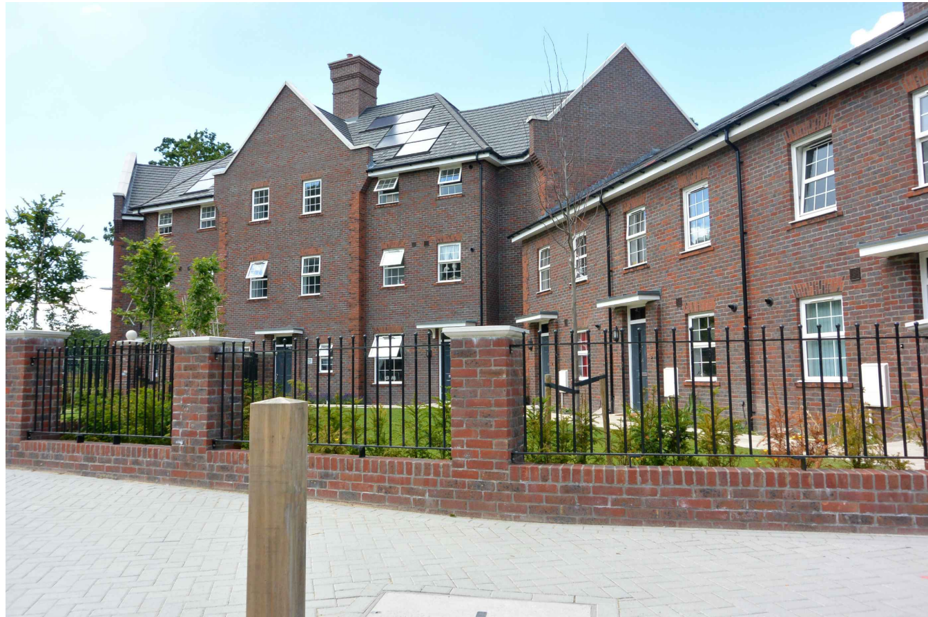
Low level railing with brick piers
