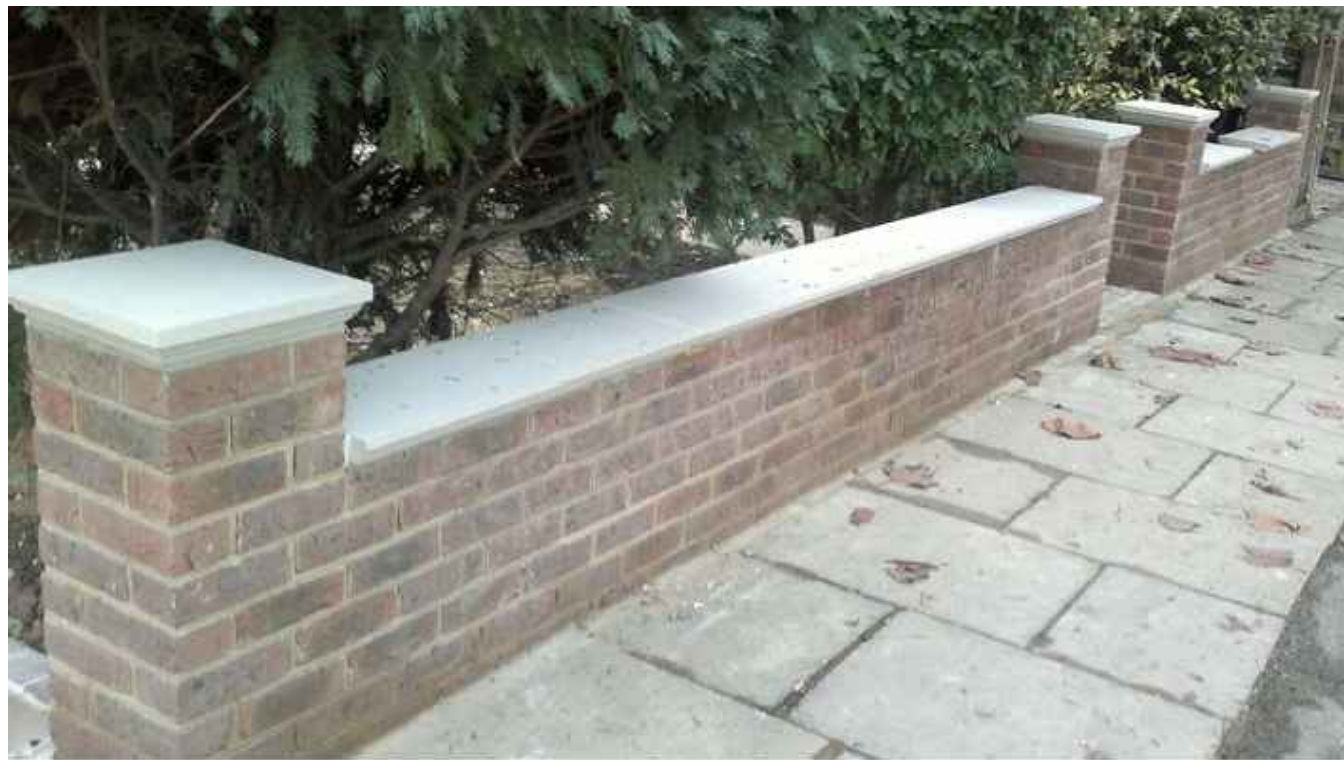
Low level wall
