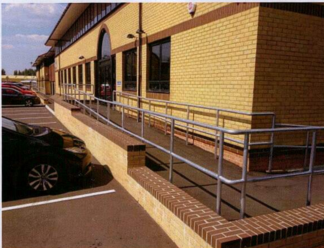
Appendix A – Figure 9: view from South-east. Ramp to be removed.
