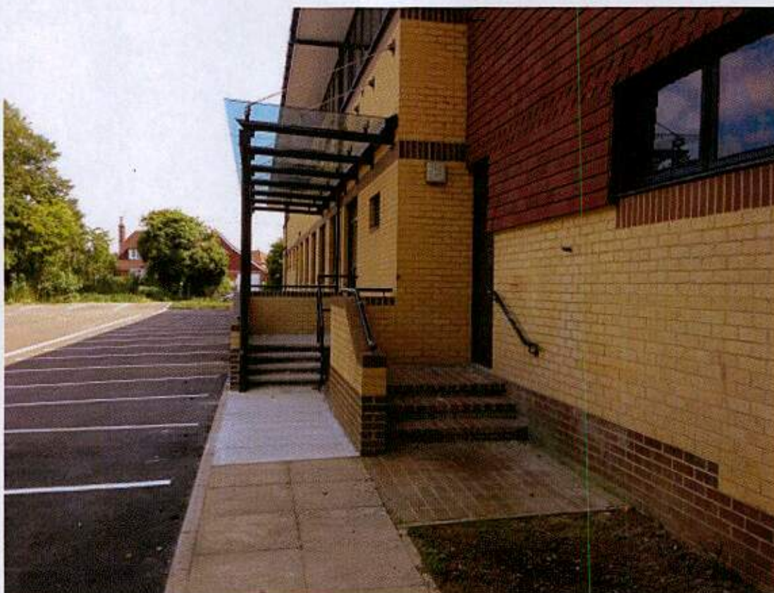
Appendix A – Figure 3: view of existing canopy and stairs. To be removed with new ramp for fire escape constructed.
