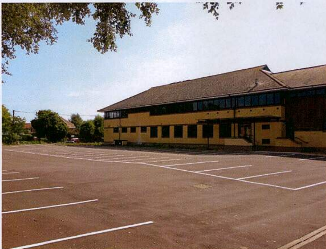
Appendix A – Figure 1: view from North showing existing car park.
