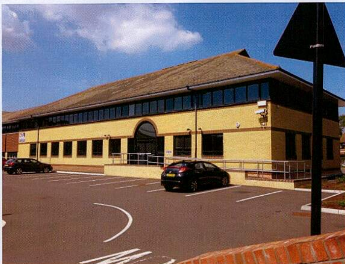
Appendix A – Figure 7: view from South-east. Access ramp to be removed.
