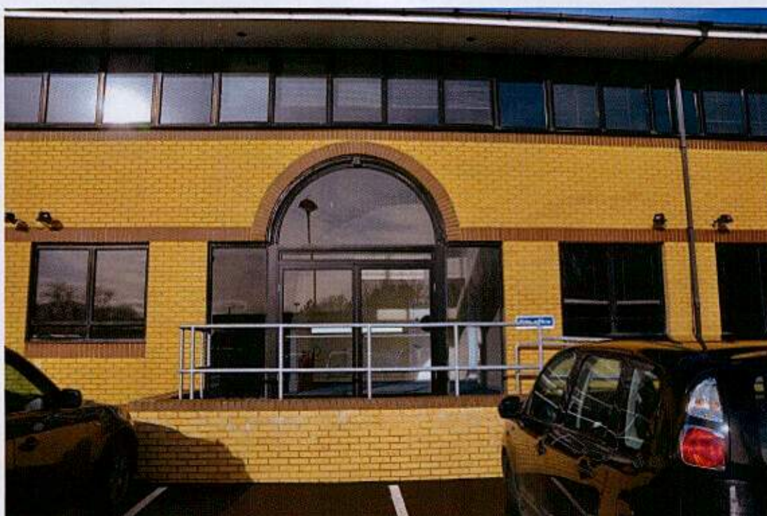
Appendix A – Figure 6: view from South of glazed door to be removed.
