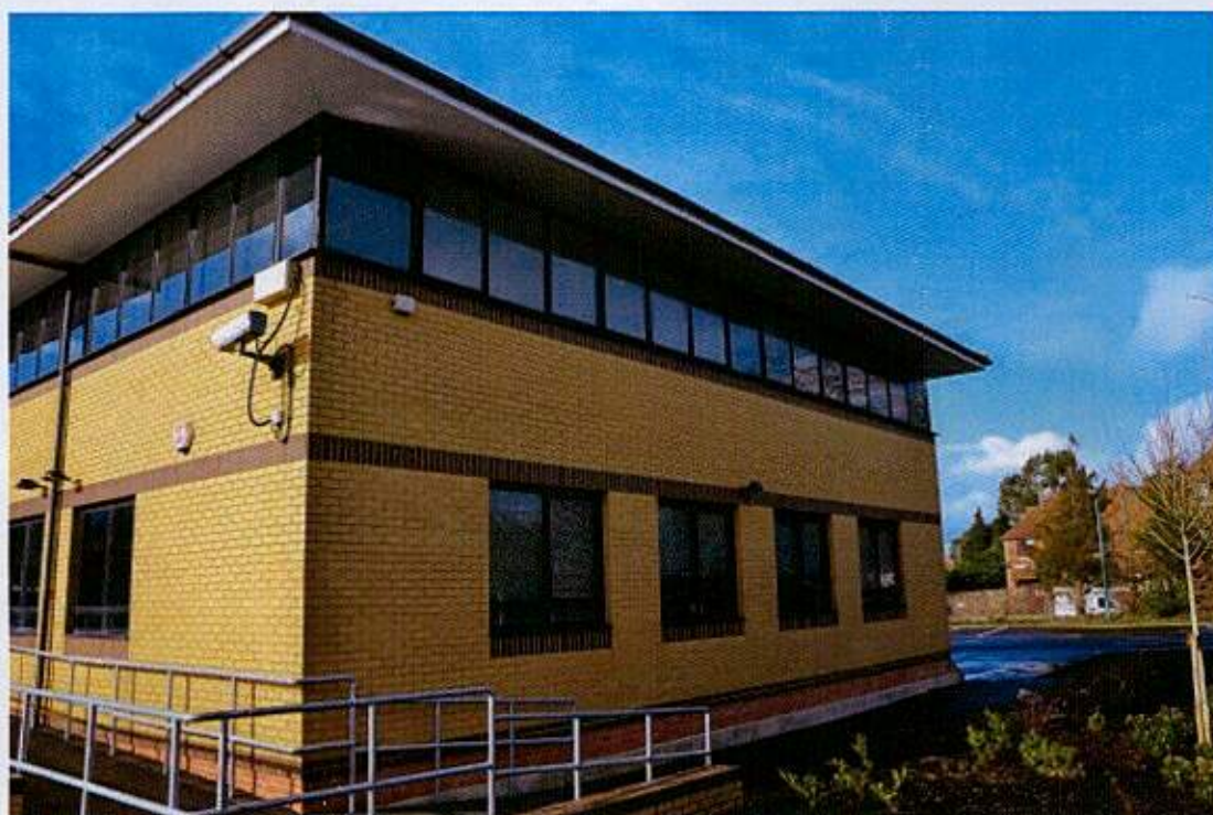
Appendix A – Figure 8: view from East. New extension to far corner.
