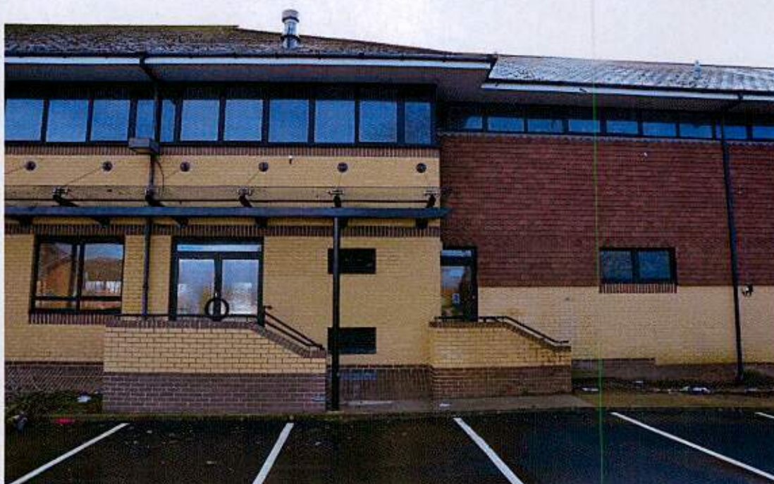
Appendix A – Figure 4: existing canopy and stairs – as Figure 3.
