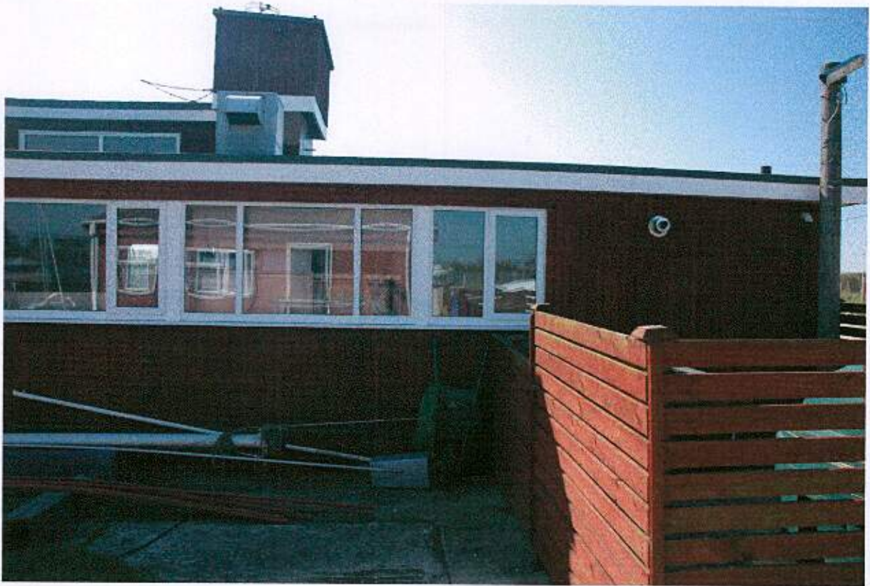
Arun Yacht Club—Main Building—North elevation (1)
