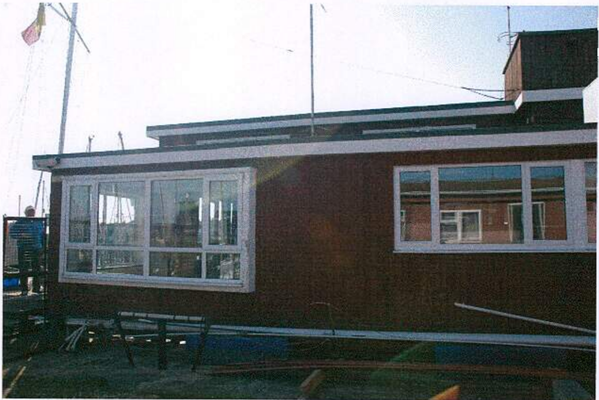
Arun Yacht Club—Main Building—North Elevation 2
