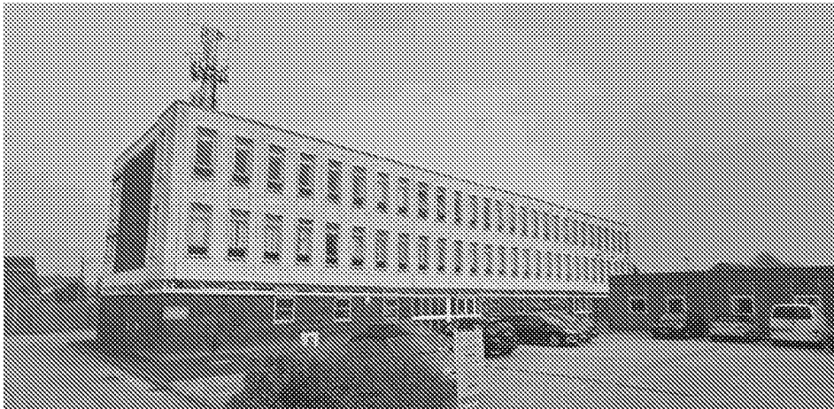
Littlehampton Police Station - 3 storey context
