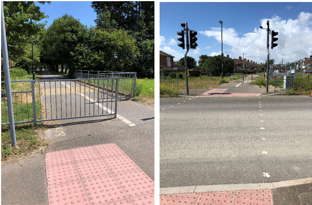
Existing Toucan Crossing on Fitzalan Road
