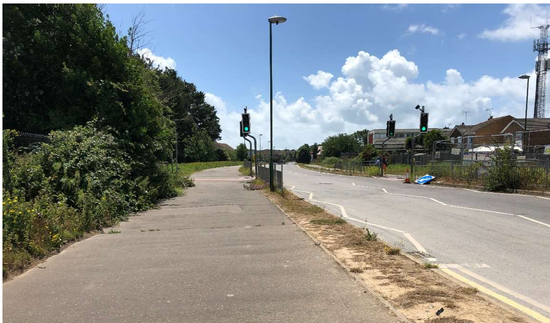
Existing Shared Pedestrian/Cycle Route on Fitzalan Road
