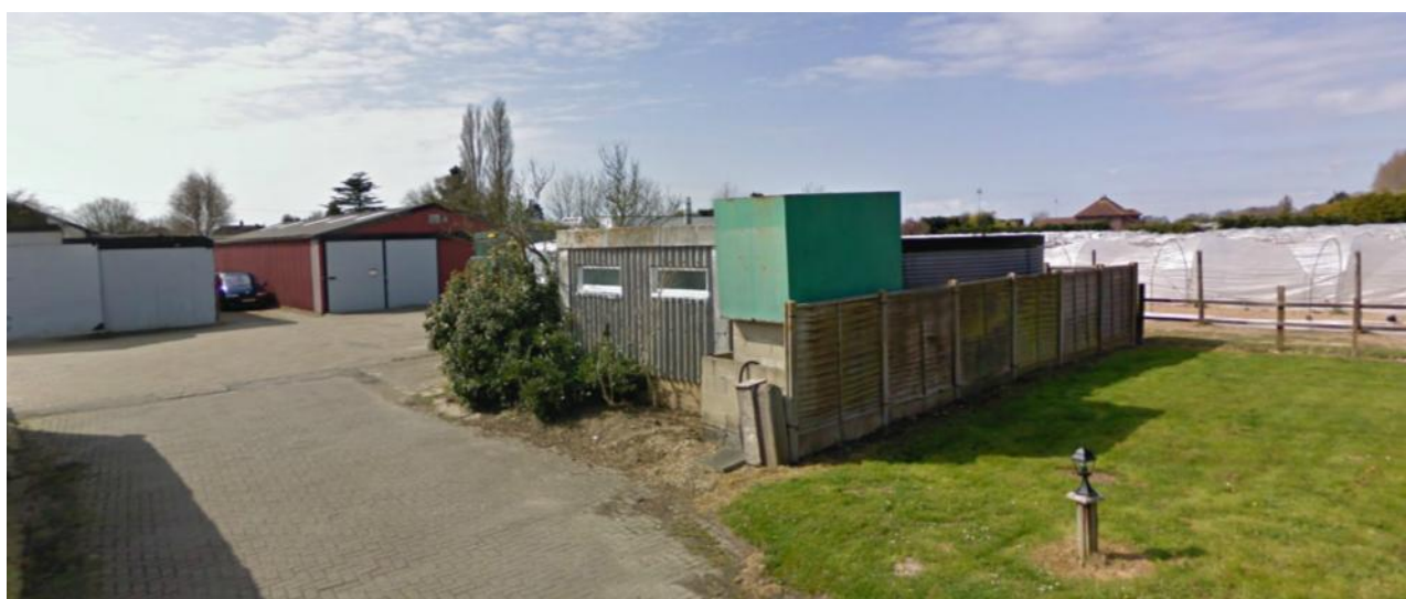
Figure 3 - Existing Buildings on Site
