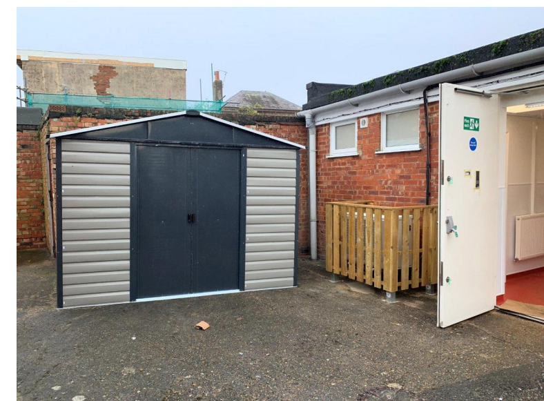
PHOTO OF METAL SHED FROM SOUTH ELEVATION
