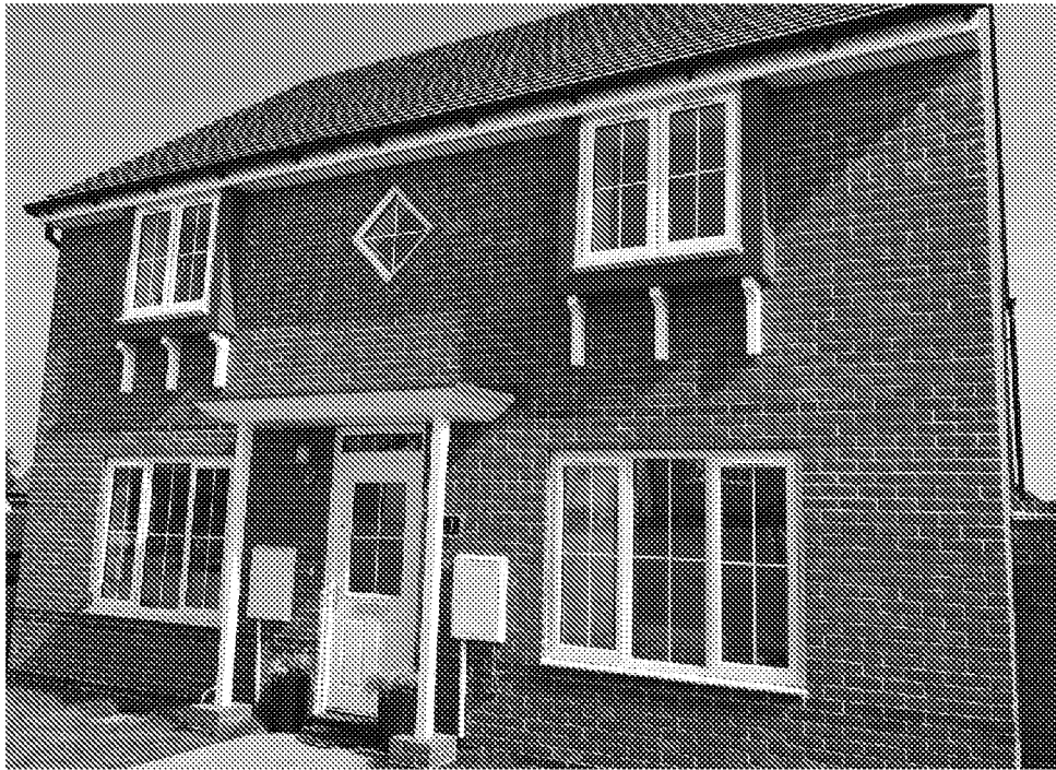
Fenestration & detailing 'constructed' image
