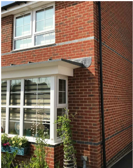
Brick/window detailing 'constructed' image
