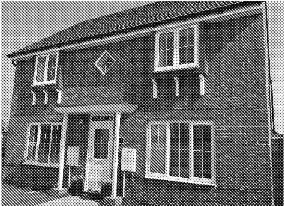
Fenestration & detailing 'constructed' image
