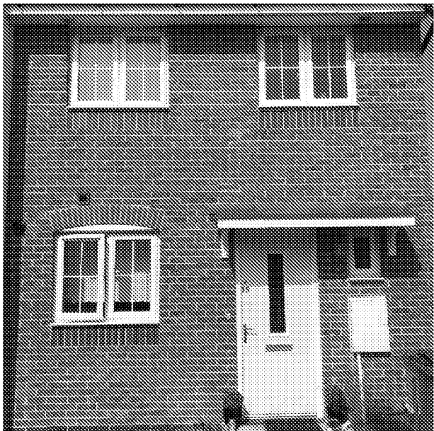
Fenestration & detailing 'constructed' image
