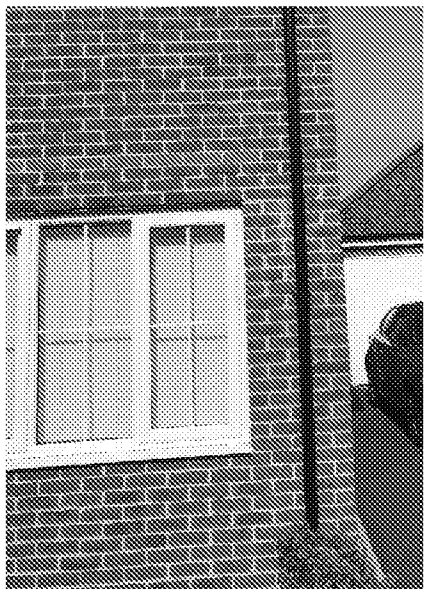
Brick detailing 'constructed' image
