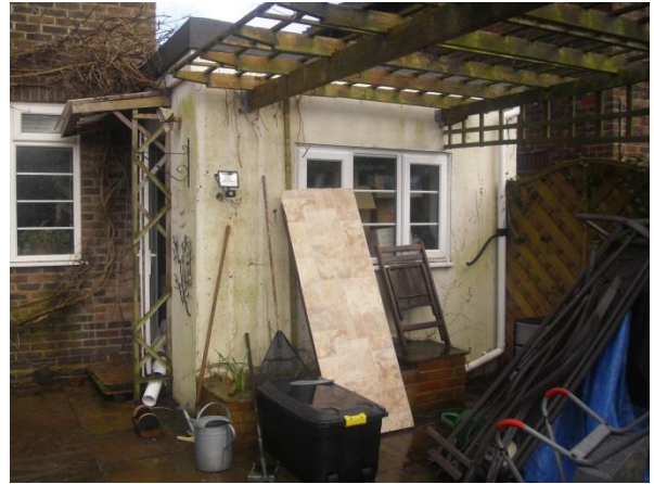
Part South Elevation from Garden.
