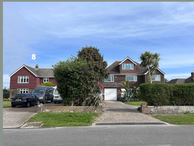
No. 8 showing adjacent property to the East
