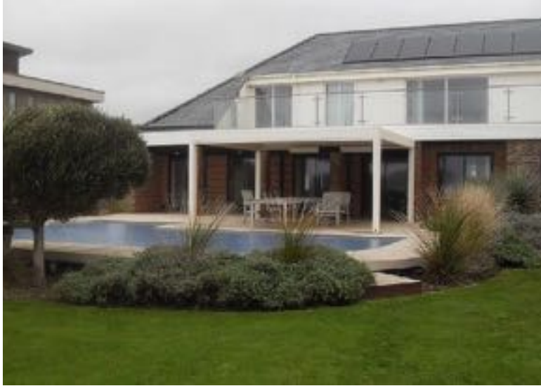
Rear Elevation from east
