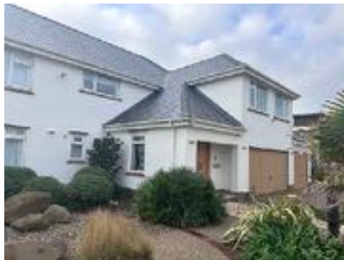
Photograph of existing front elevation looking west
