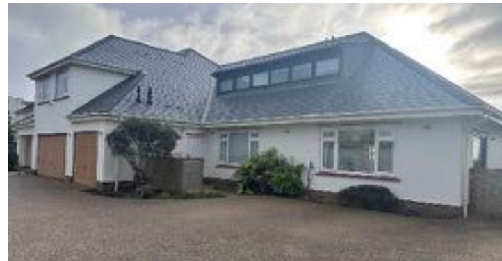
Photograph of existing front elevation looking east
