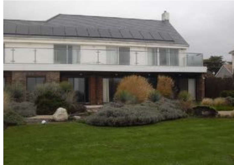
Rear Elevation from west
