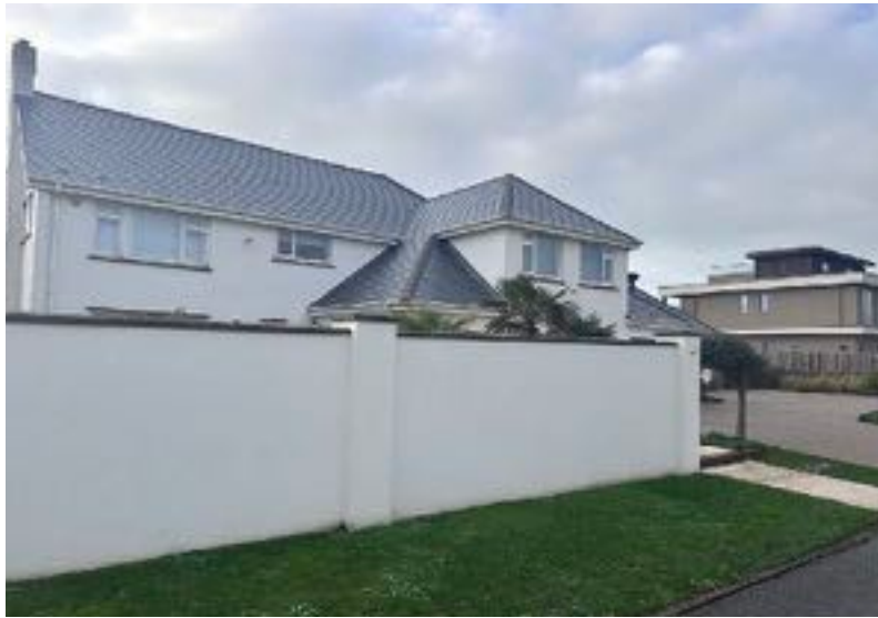
Front Elevation viewed from east
