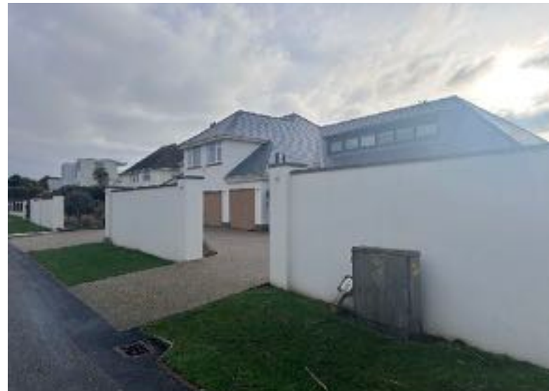
Front Elevation viewed from west
