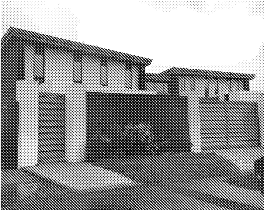
Houses within the immediate vicinity
