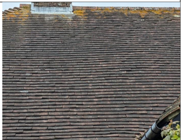
Photograph 6: Uneven roof tiles on the north elevation.
