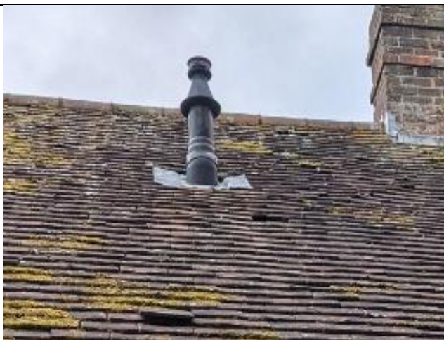
Photograph 5: Loose lead flashing around the roof vent and lifted tiles.
