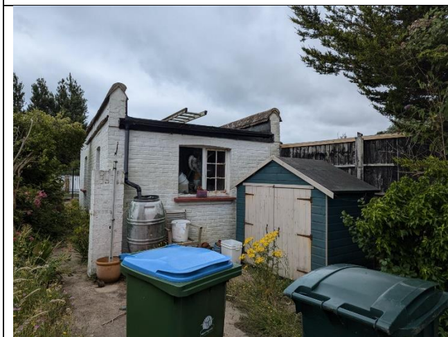
Photograph 9: North elevation of the garage showing lack of roof void.
