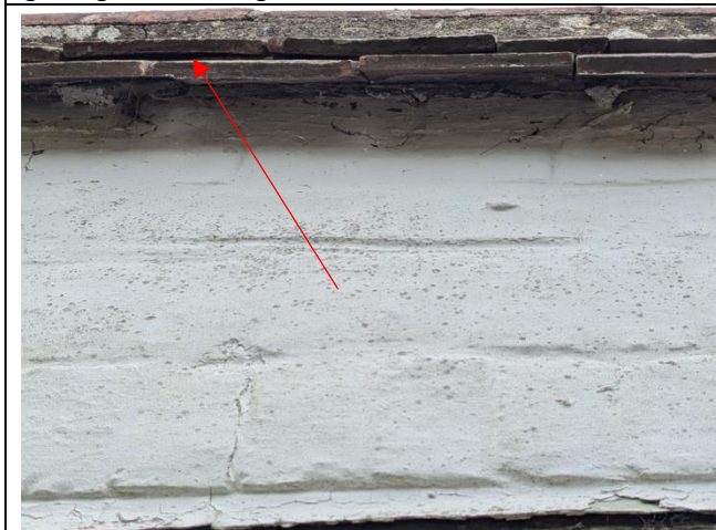
Photograph 11: A narrow gap in the decorative roof tile.
