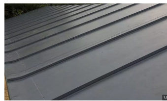
STANDING SEAM SINGLE PLY MEMBRANE
