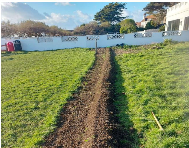
Figure 3 - Photograph of marker post and offset earth banking.
