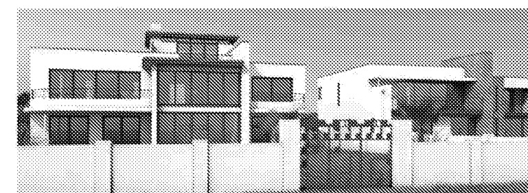
no. 69 Coastal Road (existing)
