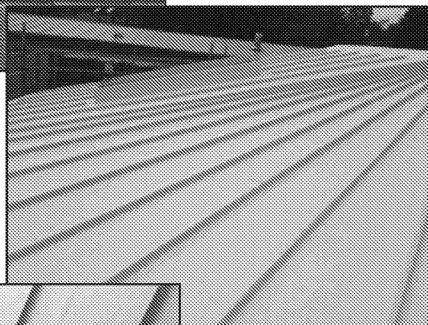
Existing warehouse conversion to domestic housing apartments. Memtec Single Ply PVC membrane roof coverings to pitched roof slopes and gutters with Memtec decarib PVC profiles roof decoration (optional).
