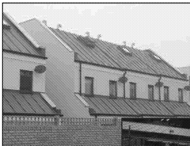
New school extension construction project. Memtec Single Ply PVC membrane roof coverings with Memtec decarib pvc profiles roof decoration (optional).
