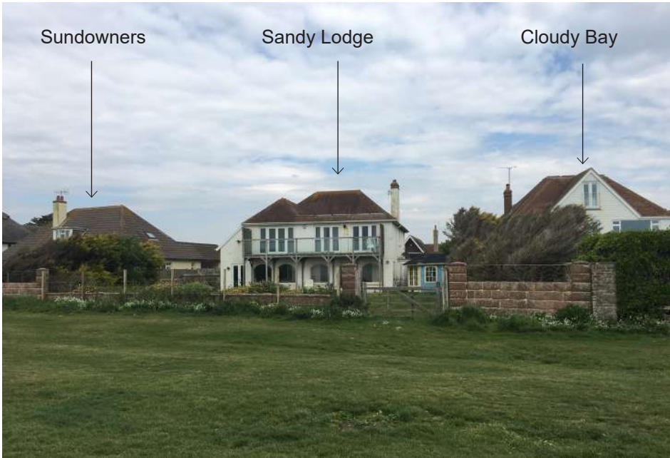
3 - Exposed southern boundary
