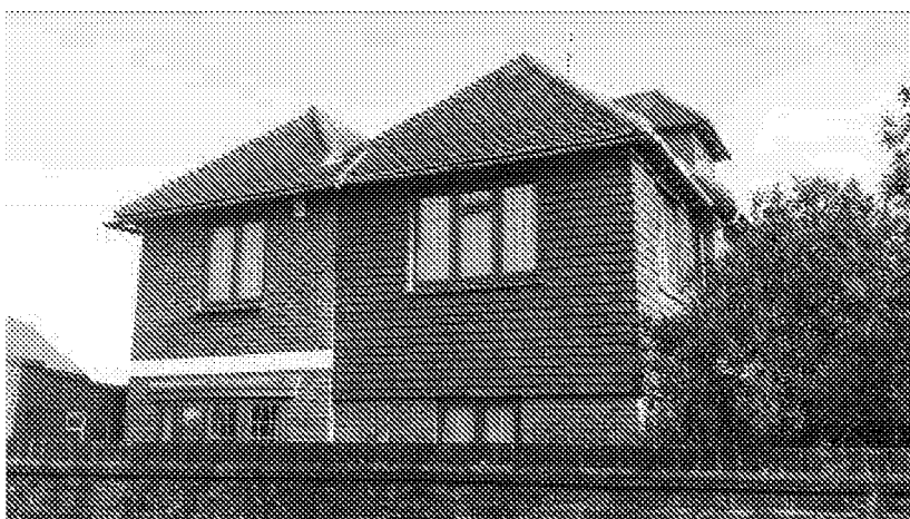
3 Storey Scea Plana viewed from Gorse Avenue
