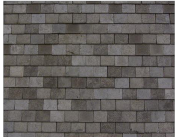
Roof: Grey slate roof tiles
