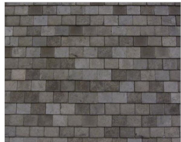
Roof: Grey slate roof tiles
