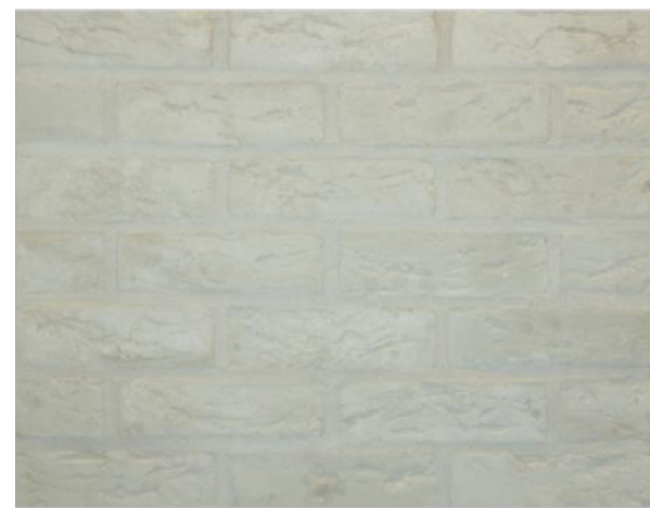
External walls: 65mm Karma White Handmade Bricks
