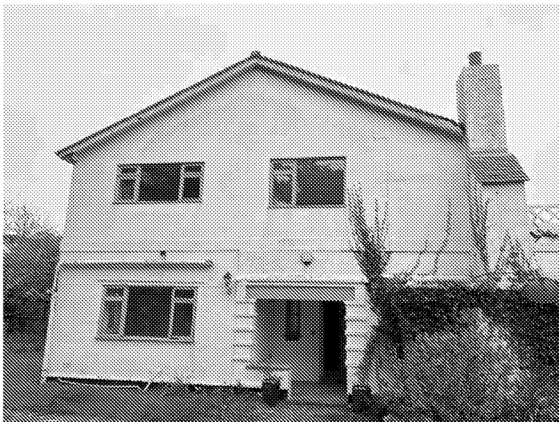
West elevation of Panorama – front entrance
