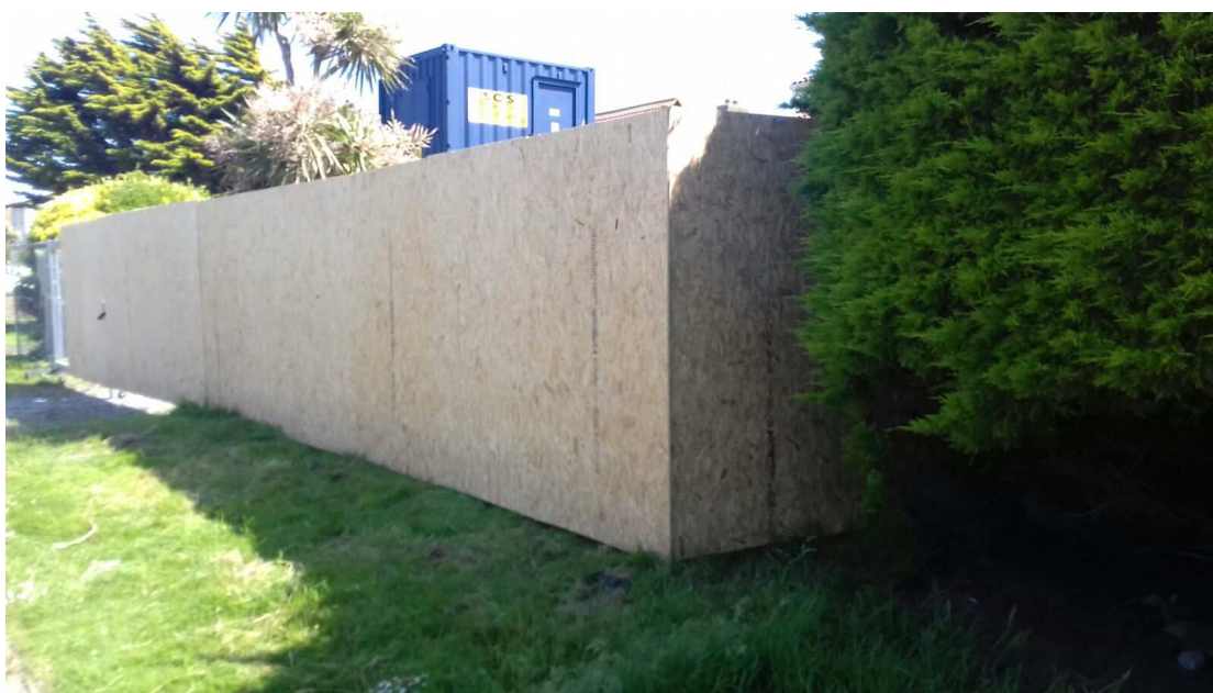
Figure 4 – La Casa North site boundary with hoarding fence
