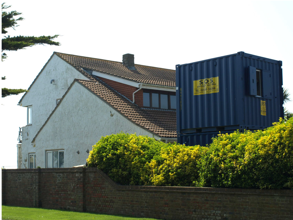
Figure 1 - La Casa viewed from Northeast
