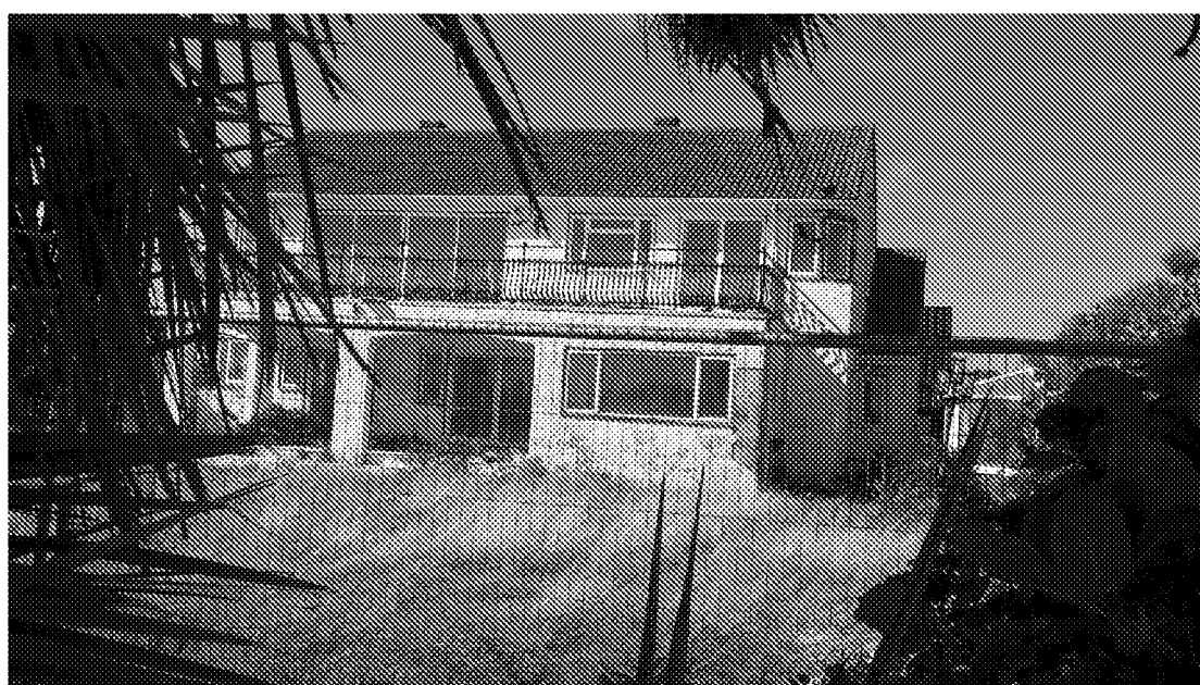
Figure 8 - La Casa viewed from the Green Sward (South Elevation)
