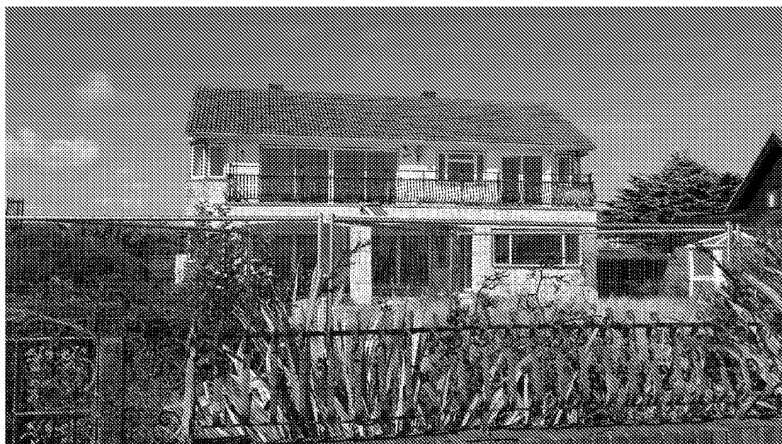
Figure 7 - La Casa viewed from the Green Sward (South Elevation)
