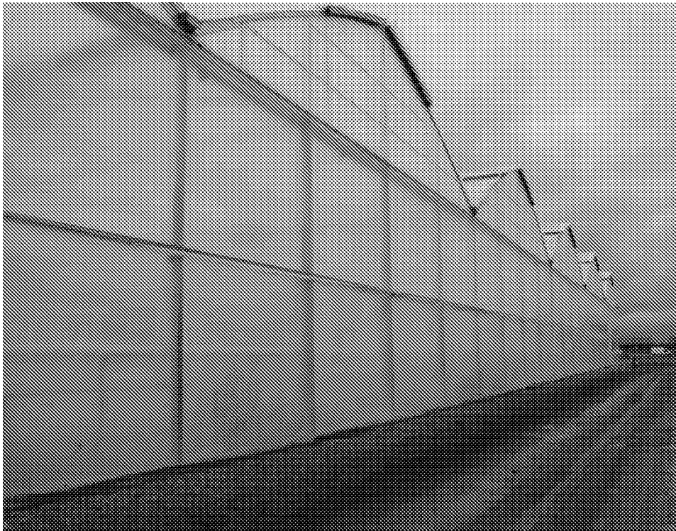
Site Photograph A. Old glasshouse type structure, but with looser plastic sheeting covered frame in place of glass type, located to the south west of the Site.
