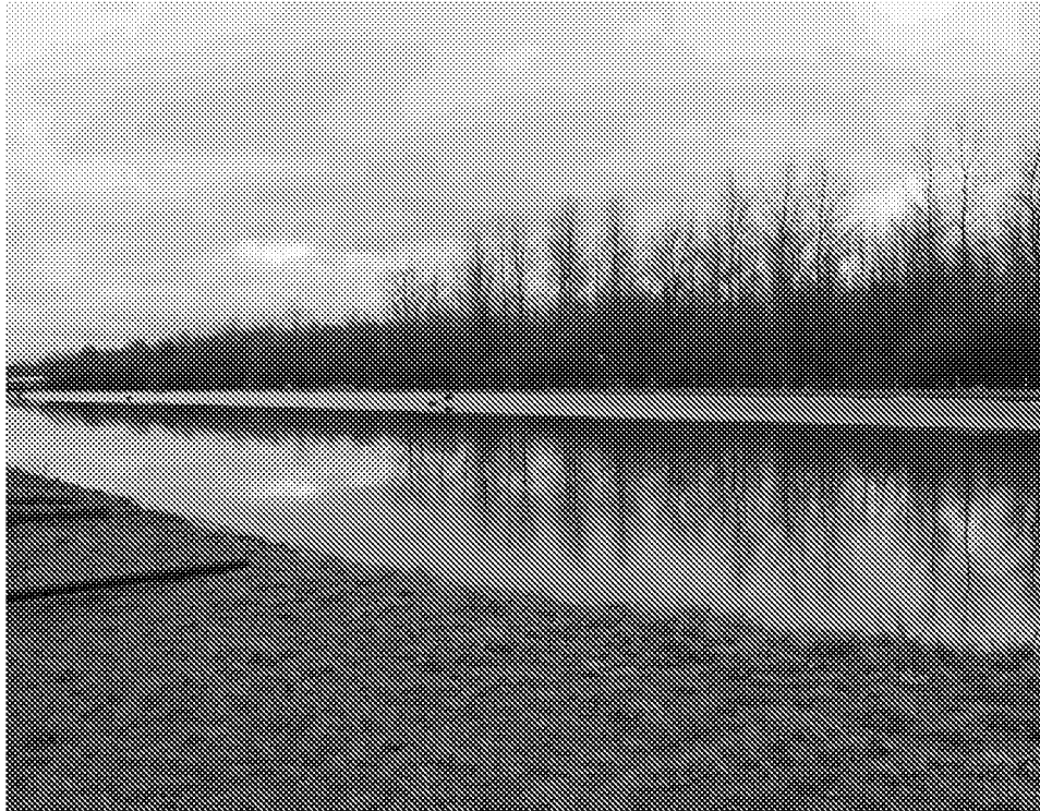
Site Photograph E. Water storage reservoir to the north of the newly built galsshouse to the west of the Site, with railway line and tree belt beyond.
