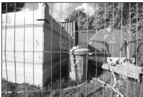
Photo 46: Where fuel or other chemical are stored on site, it is now standard practice to have emergency spillage kits available to restrict the environmental impact of accidents.
