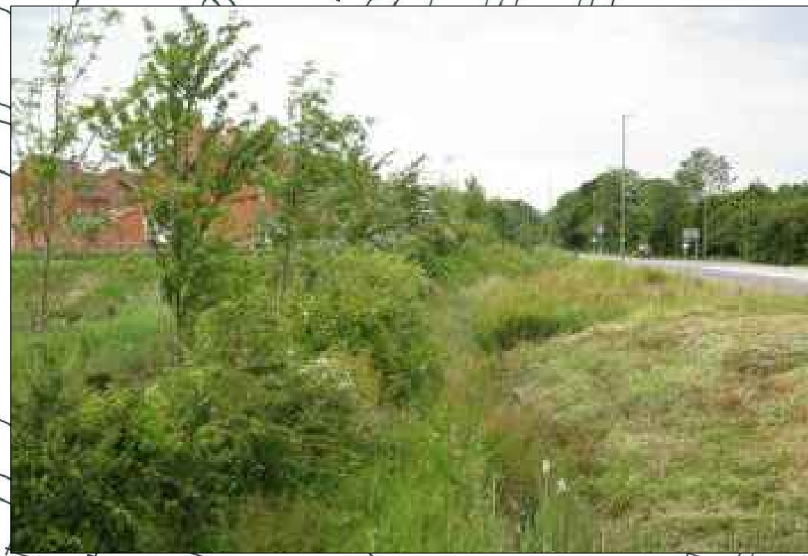
PHOTOGRAPH OF TYPICAL DRAINAGE SWALE
