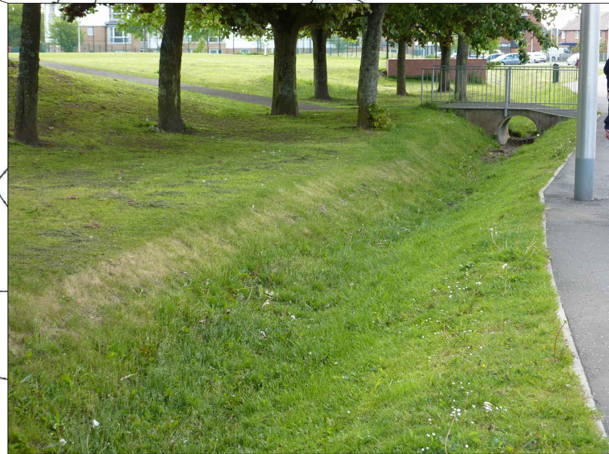
PHOTOGRAPH OF TYPICAL DRAINAGE SWALE
