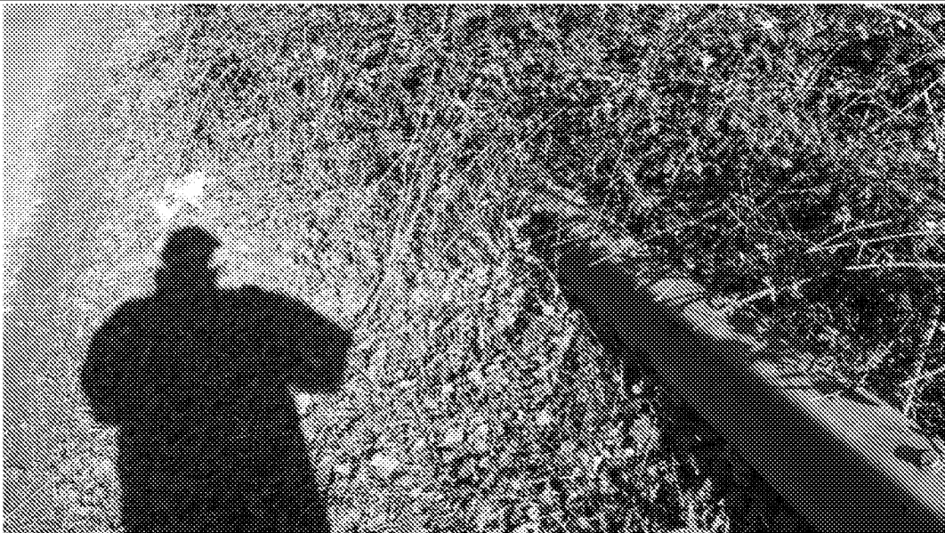
Photo B Existing damaged VRS non-compliant on east side of Ford Road
